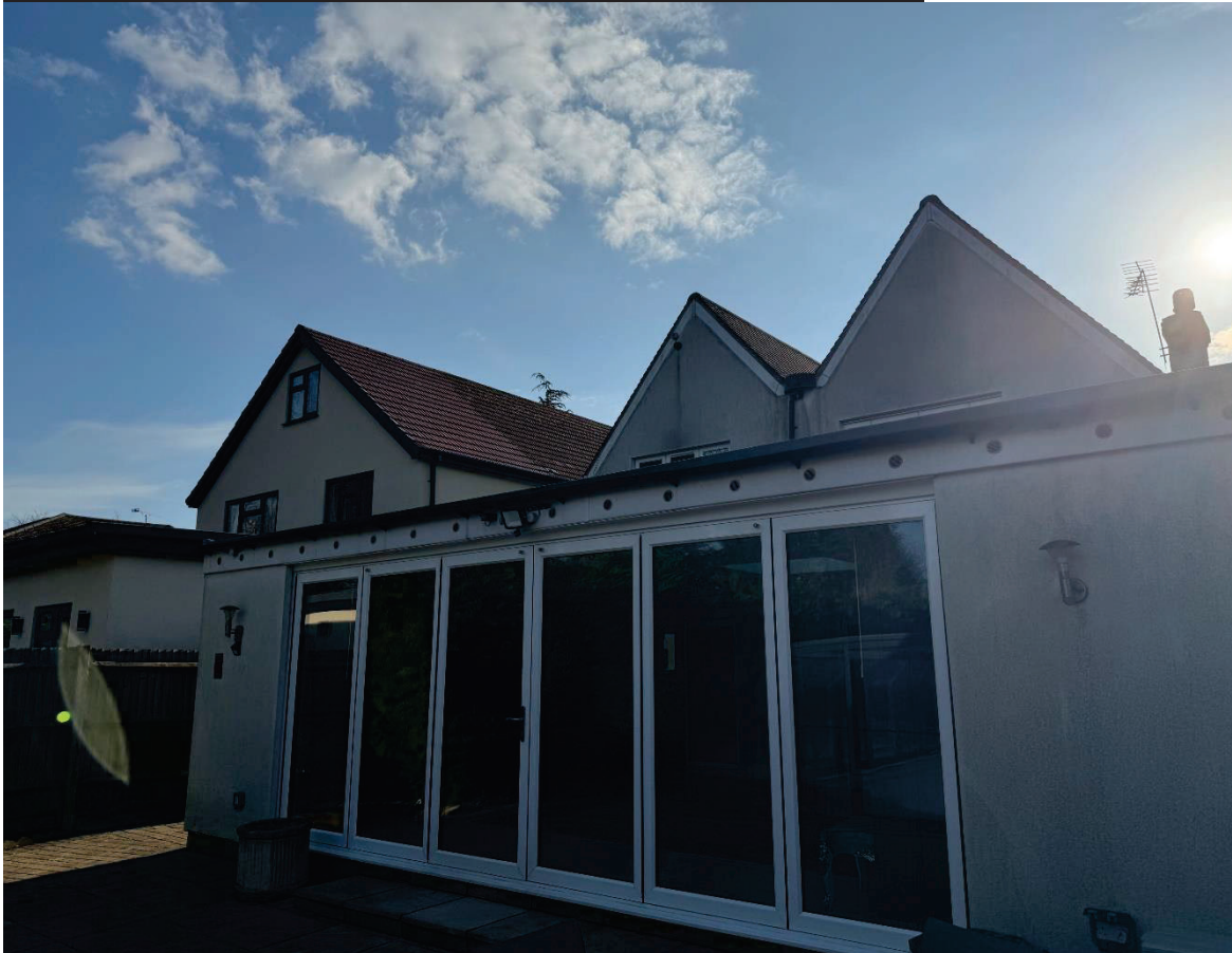
Figure 8 – Rear view of neighbour No.36 from application site
