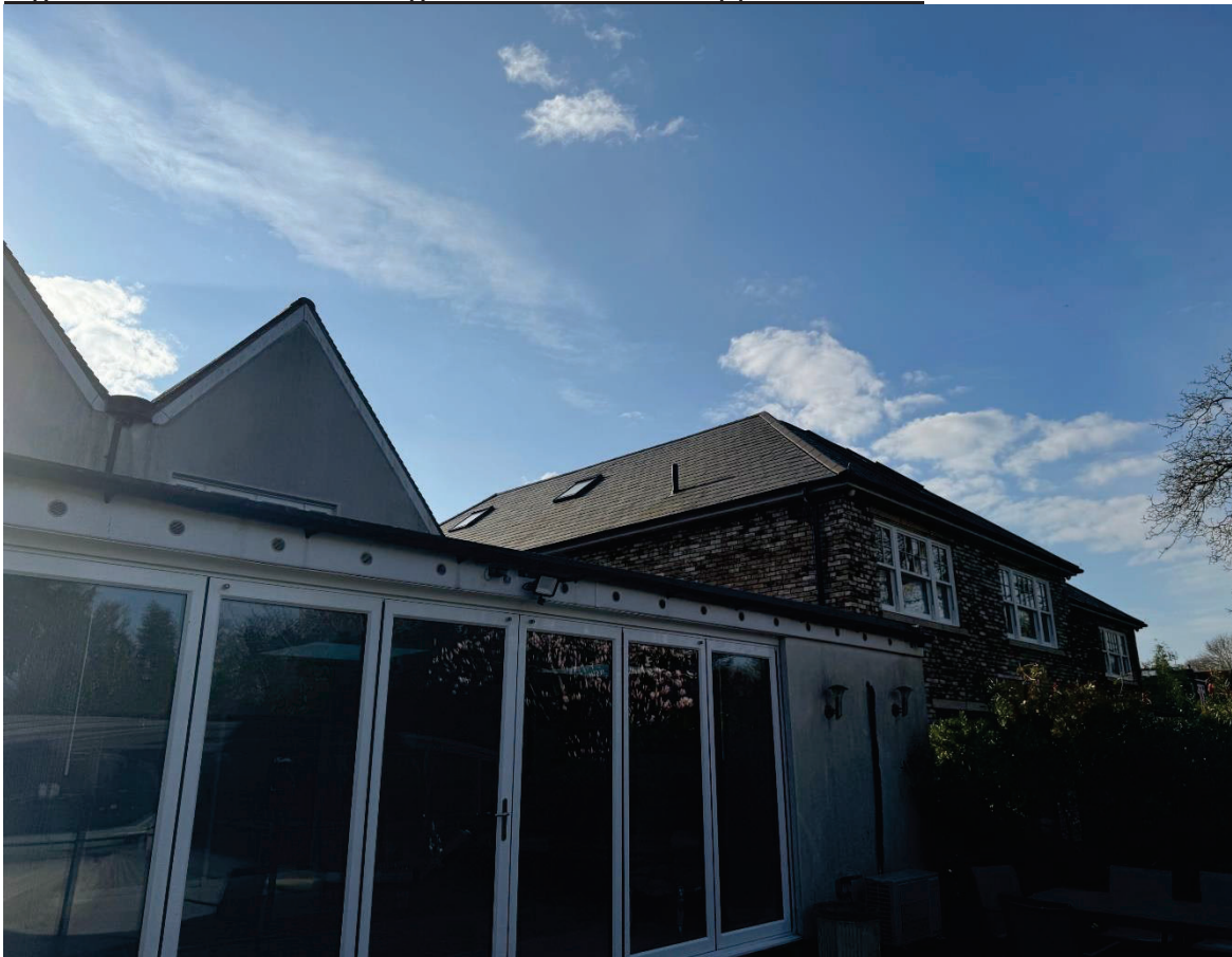
Figure 7 – Rear view of neighbour No.40 from application site
